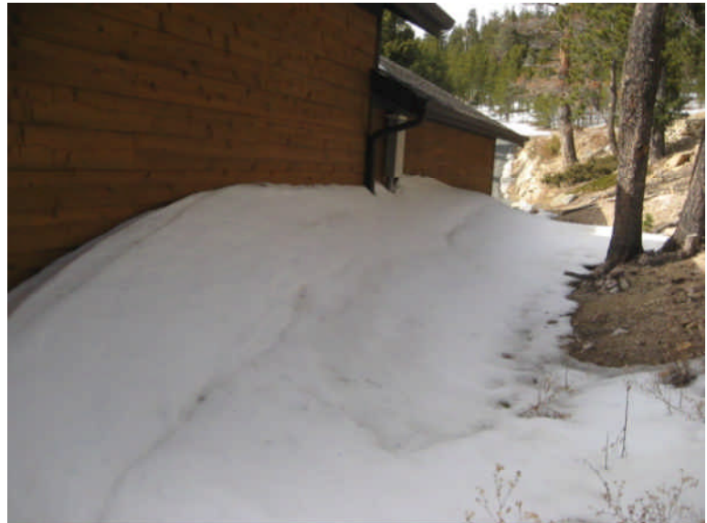
Unable to fully view due to snow cover.
